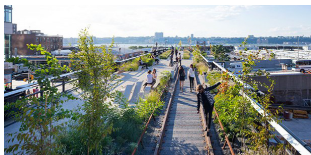
Figure 30: Highline, New York - revitalisation of an elevated disused rail line into an active transport route and major tourist attraction.
